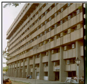
Coolers in Multi- Storied buildings in urban areas
